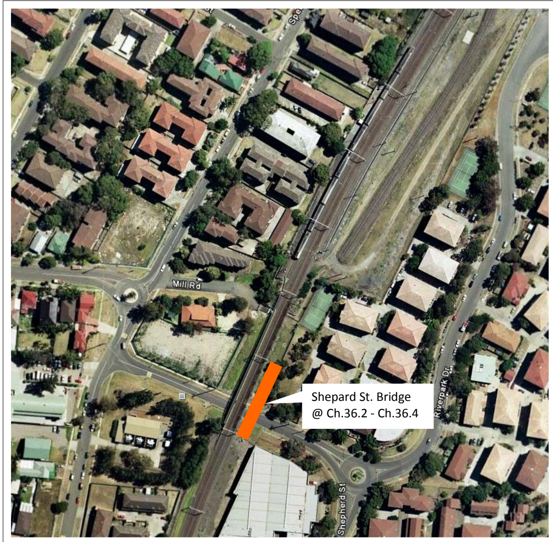
Shepard St. Bridge - BR2 @ Ch.36.2 - Ch.36.4
