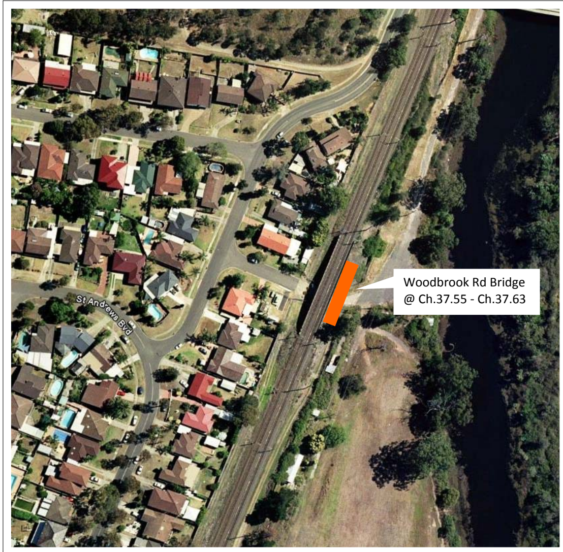
Woodbrook Road Bridge - BR2 @ Ch.37.55 - Ch.37.63
