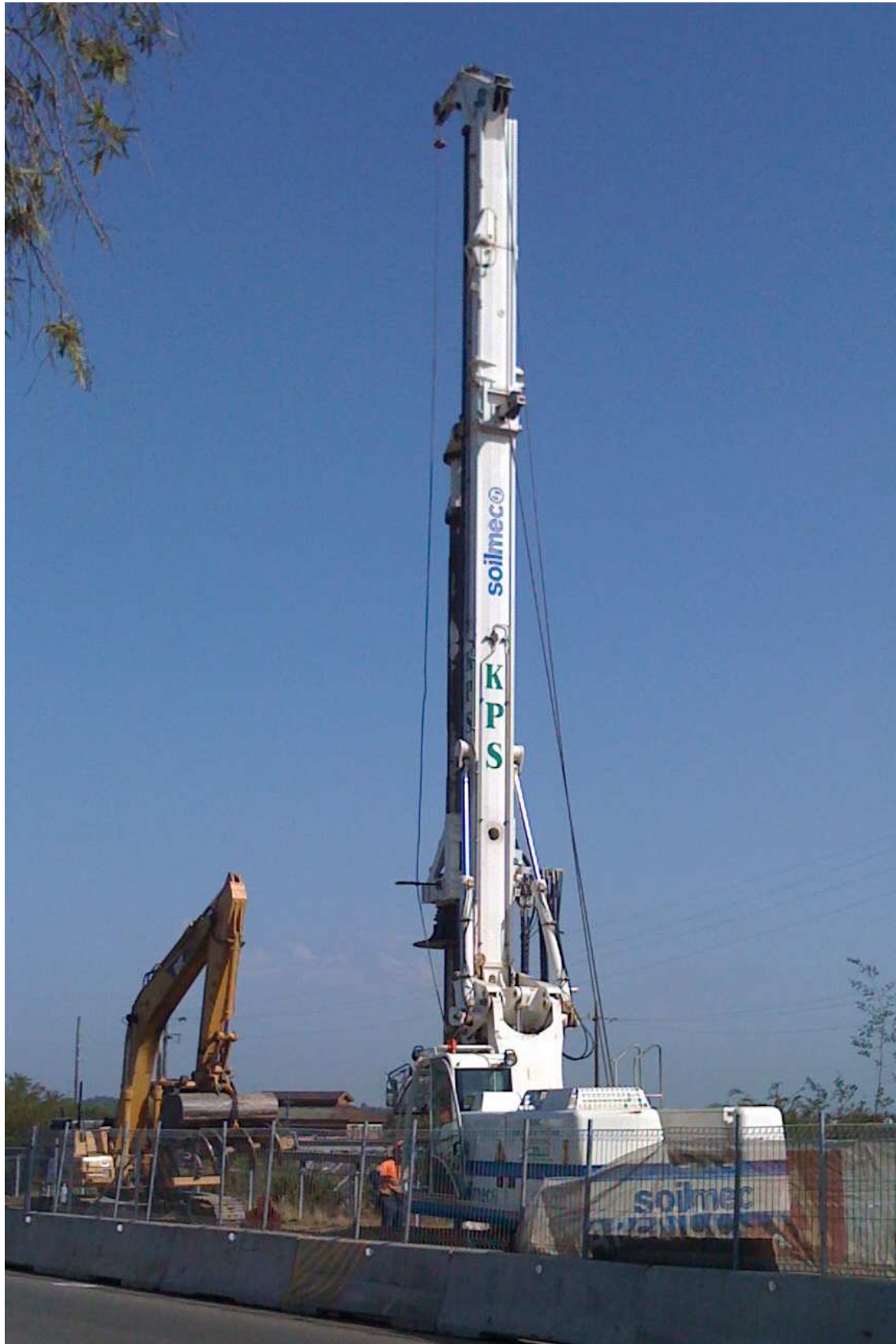
Photograph of drilling rig Soilmeco SR-30.
