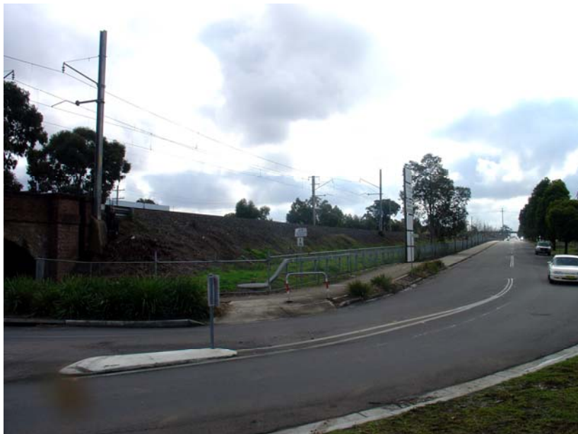
Photograph 5.1 View of western side of Broomfield Street, near the underbridge
